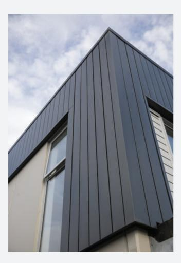
**DESIGN CONSIDERATIONS** - Interlocking Panels can be installed horizontally, vertically or diagonally. A specific feature of this cladding is that it is installed from top to bottom when used horizontally. Special attention is needed to position any penetrations in the walls so that they are aligned with the recessed joints - horizontally and or vertically.
